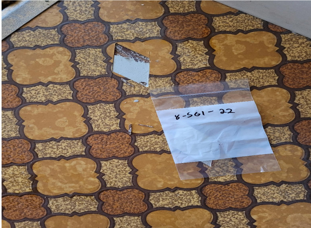
Photo 3: View of positive vinyl sheet flooring in building 211 2 nd floor north end apartment kitchen.
