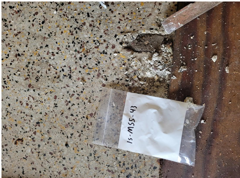
Photo 6: View of positive terrazzo flooring in building 213 1 st floor office space.
