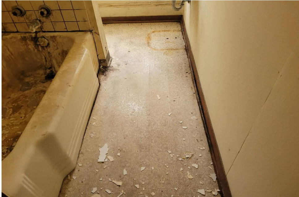
Photo 5: View of positive vinyl sheet flooring in bathroom of building 213 2 nd floor apartment.
