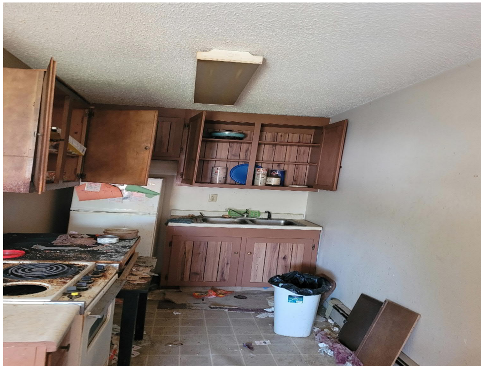
Photo 4: View of positive vinyl sheet flooring 2 layers in building 211 2 nd floor south end apartment kitchen.
